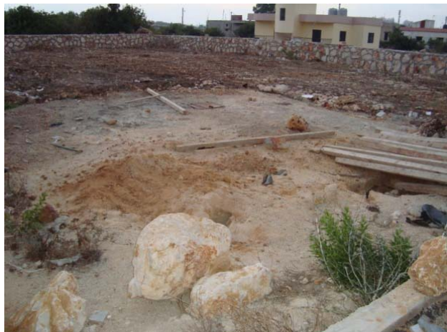
Construction of olive press in Yarin
