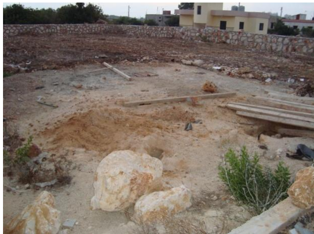
Construction of olive press in Yarin
